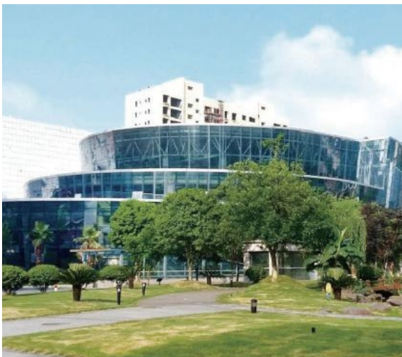
湖南湘西自治州烟草公司体育馆 Gymnasium for the Tobacco Company of Xiangxi Prefecture, Hunan
